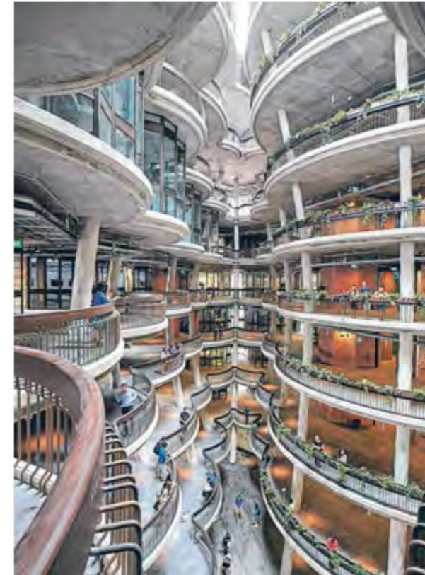
The $45 million learning hub unveiled by NTU in March this year. Composed of 12 towers of stacked, rounded rooms, the hub is aimed at supporting the university's "flipped classroom" approach. PHOTO: HUFTON AND CROW
