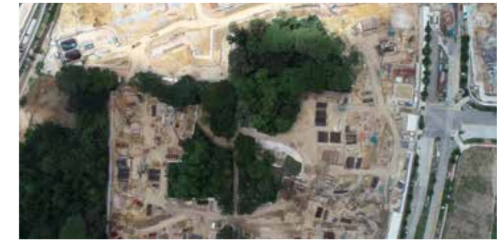
Plot 1 construction progress as of March 2020
