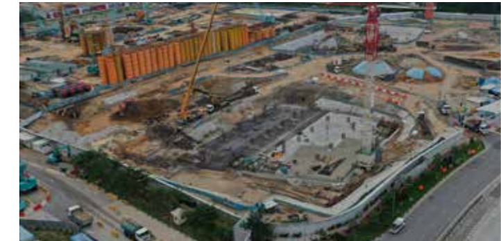
Plot 2 construction progress as of March 2020
